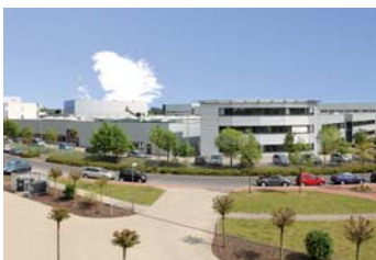
MEISINGER Headquarters Neuss, Germany
